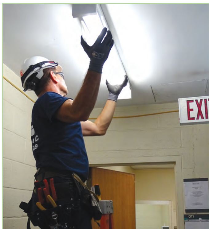
FSG ELECTRICIAN RETROFITTING A FIXTURE FROM FLUORESCENT TO LED.
