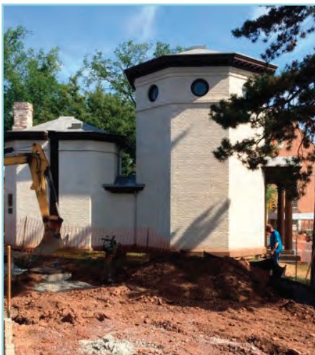
SCHANCK OBSERVATORY IN JULY 2016, WITH DRAINAGE IMPROVEMENTS IN PROGRESS.
