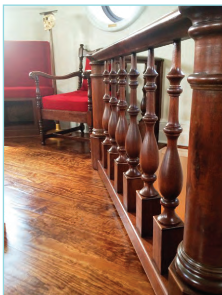
RECREATED FLOORING AND RESTORED HANDRAIL ARE AMAZING.
