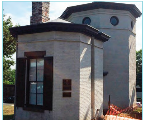
THE OLD WORKROOM, NOW RESTORED AS A LOUNGE. COATED BRICKWORK REPLICATES THE ORIGINAL.
