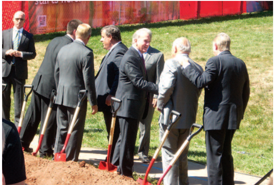
NEW JERSEY GOVERNOR CHRIS CHRISTI AND RUTGERS PRESIDENT ROBERT BARCHI TAKE PART IN THE COLLEGE AVENUE INITIATIVE GROUNDBREAKING
