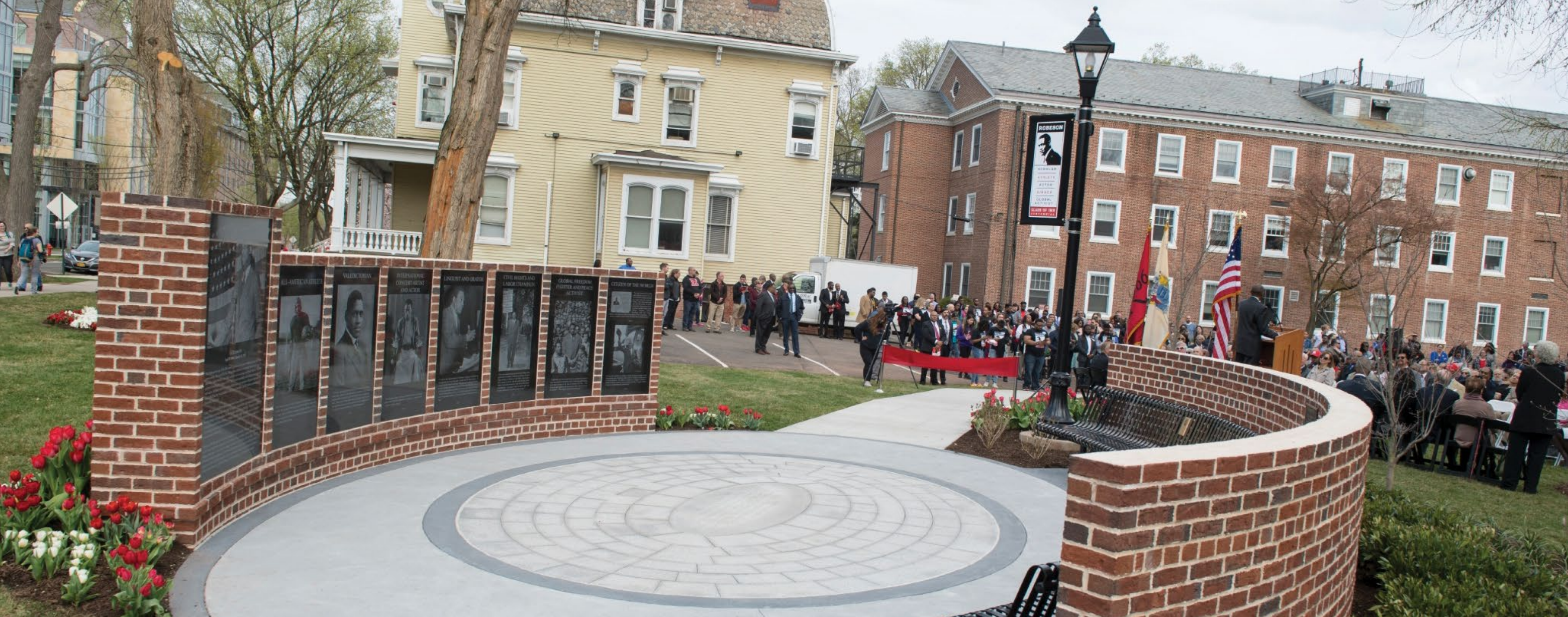
The outdoor plaza, which features eight black granite panels detailing the story of Paul Robeson's life, stands in a prominent location next to the Voorhees Mall on the College Avenue Campus.
