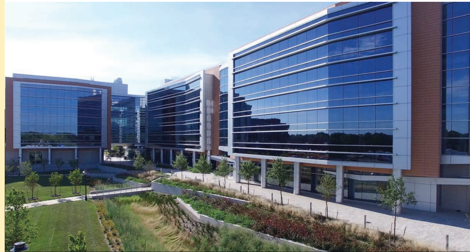
Above: State-of-the-art Chemistry and Chemical Biology Building opened in September 2018. PHOTO COURTESY OF RUTGERS UNIVERSITY
